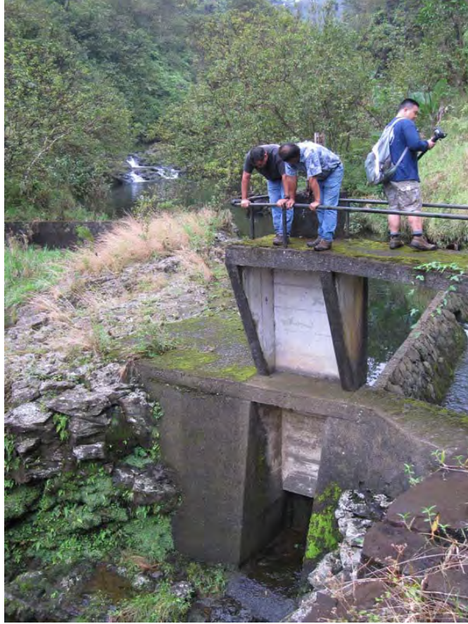
View of diversion and cascading fall in the background
