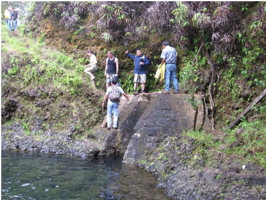
Diversion intake to left of waterfall
