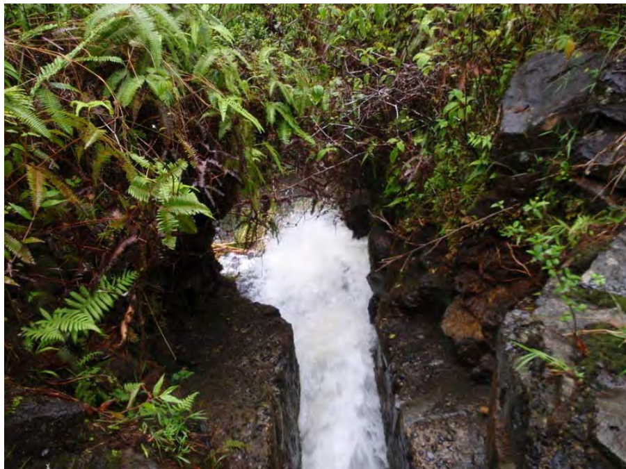
Flume from control gate into stream (gh002d-021p-041012)
