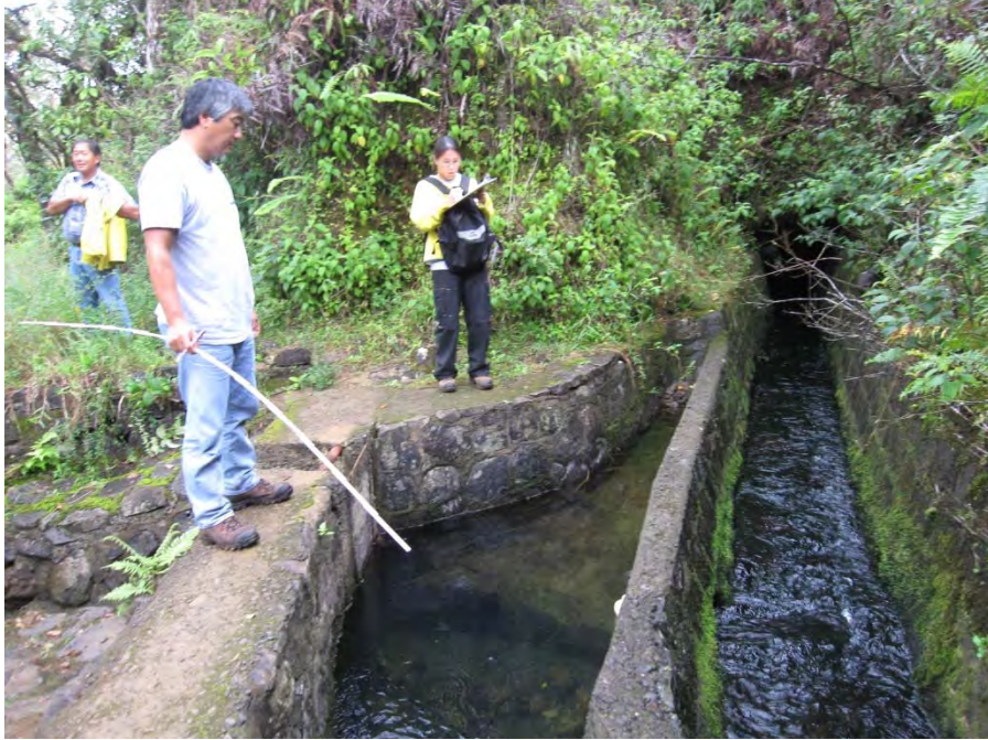
Diversion ditch connected to intake and just above site#4. Ditch release door and channel to the left of Lance's feet.
