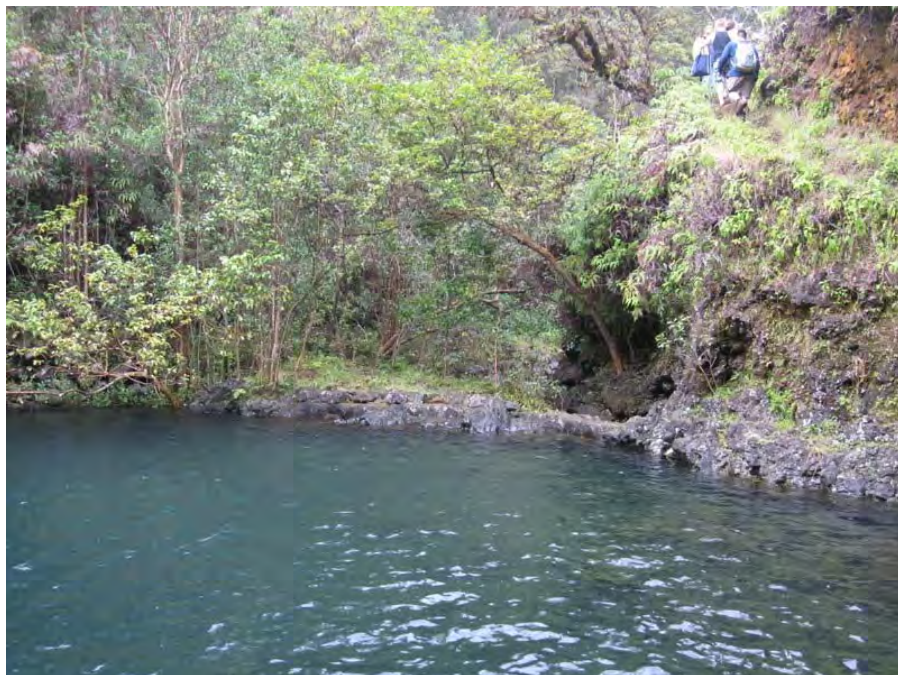
Dam wall in plunge pool downstream view
