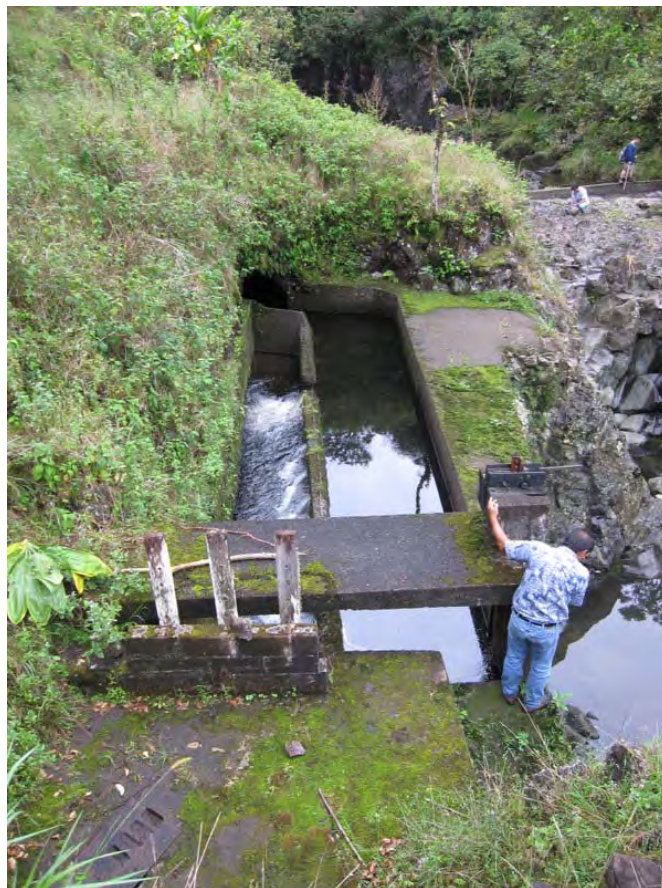
Diversion view from bridge
