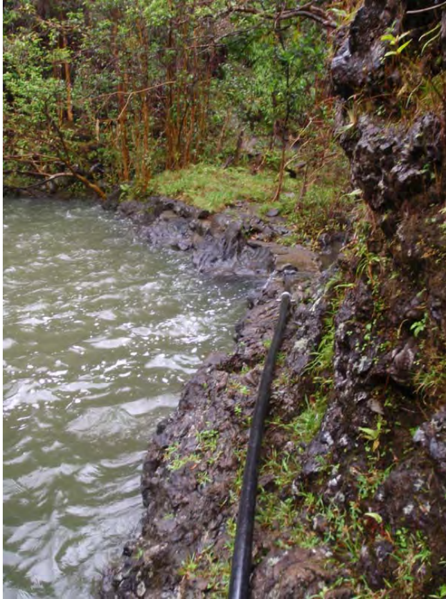
Pipe to dam (gh002d-017p-041012)
