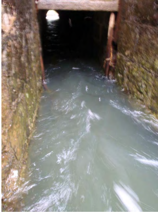
Intake tunnel (gh002d-019p-041012)
